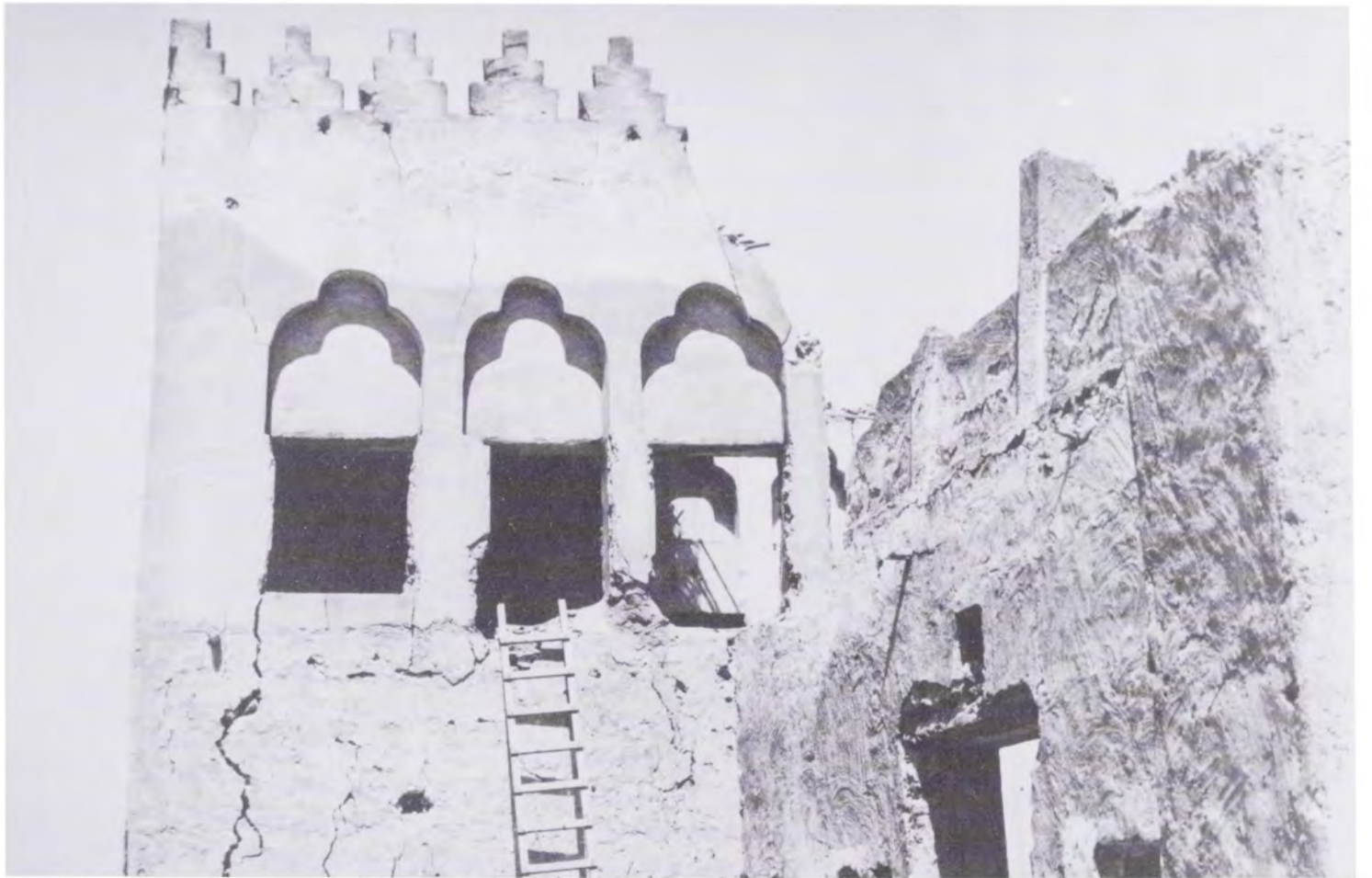
(Fig. 19) : Outer Walls of Sheikh Ali Bin Abdullah's residence before restoration.
